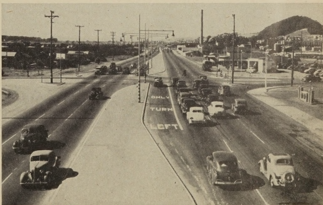
An intersection in an outlying area, with added turning lanes for left-turn movements and separated turning lanes for right-turn movements.
